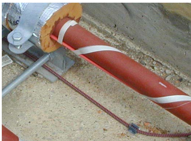
TraceTek TT5000 cable clipped to the base of the concrete trench close to the pipe, prior to the insulation being fitted.
