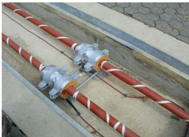
TraceTek TT5000 cable clipped to the base of the concrete trench close to the pipe, prior to the insulation being fitted.
