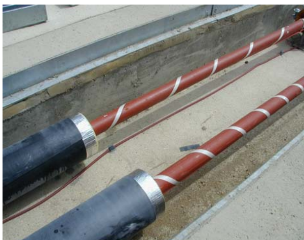
TraceTek TT5000 cable can be seen positioned below the pipes
