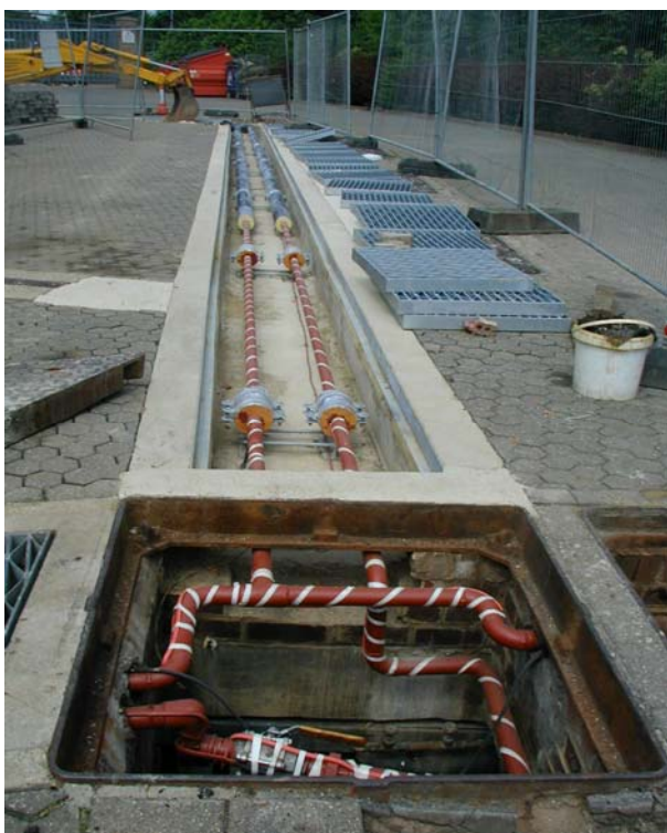
TraceTek TT5000 cable clipped to the base of the concrete trench close to the pipe, prior to the insulation being fitted.
